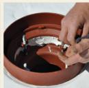
4. Seal free edges of membrane with urethane sealant.
